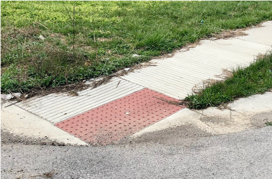
figure 6: ADA compliant curb ramps
